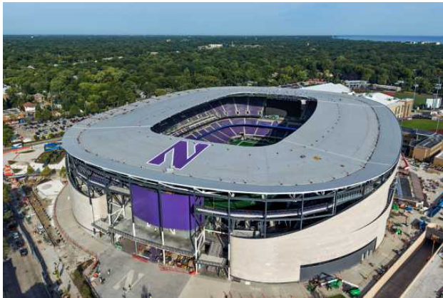
Top: Pat Ryan Jr., CEO of Ryan Sports Development, who is leading the development of the stadium, stands on the 50-yard line at Northwestern University's new Ryan Field on Monday in Evanston. It is still under construction and officially opens Oct. 2.
